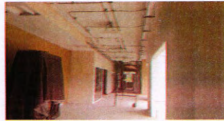
Fachada interior pasillo frontal, CURLP
