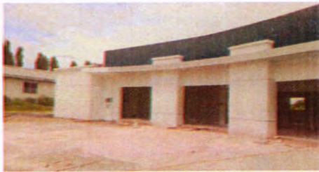
Fachada frontal, CURLP
